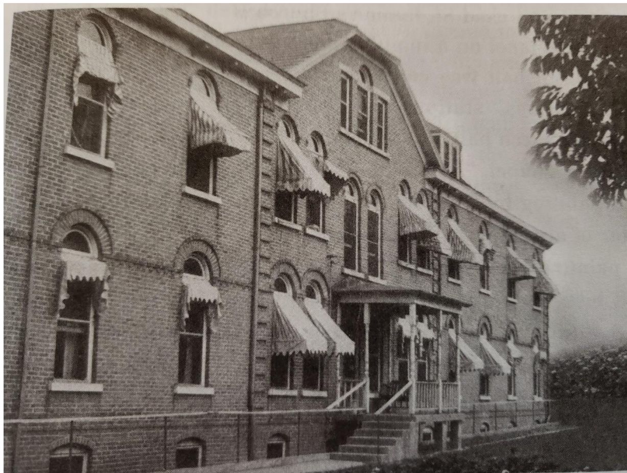
1906 Hospital Building Addition, West Side.
