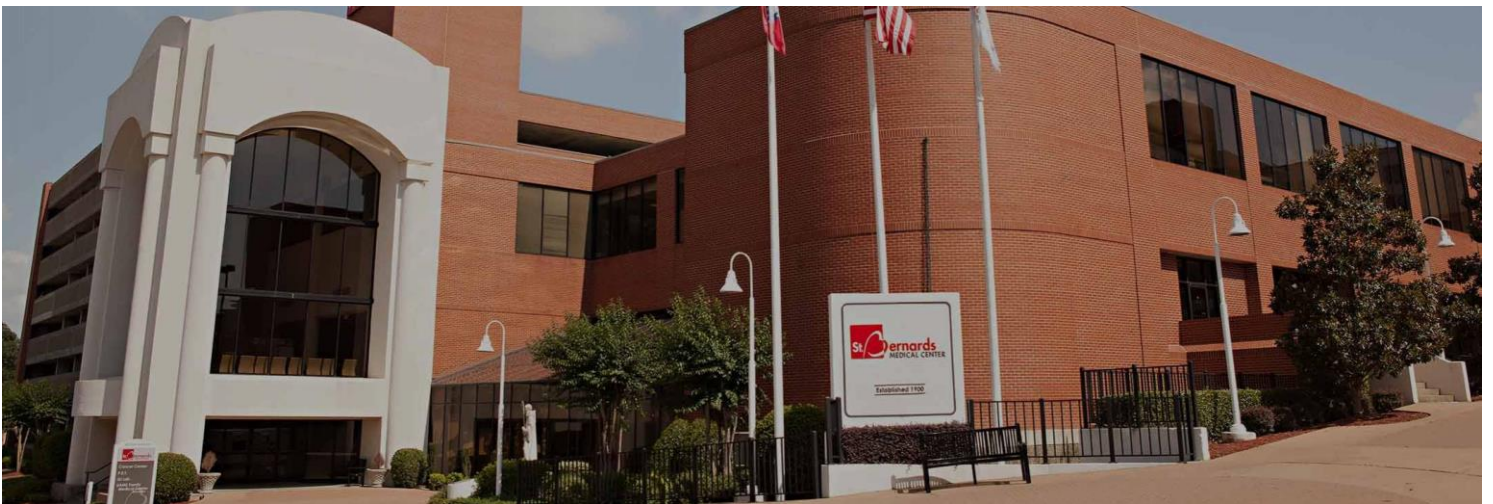
Ben E. Owens Cancer Treatment Center, north side View is southeast from E. Jackson Ave Picture Source: stbernards.info
