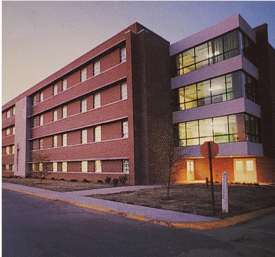
St. Bernard's Hospital, East Wing, facing south.
