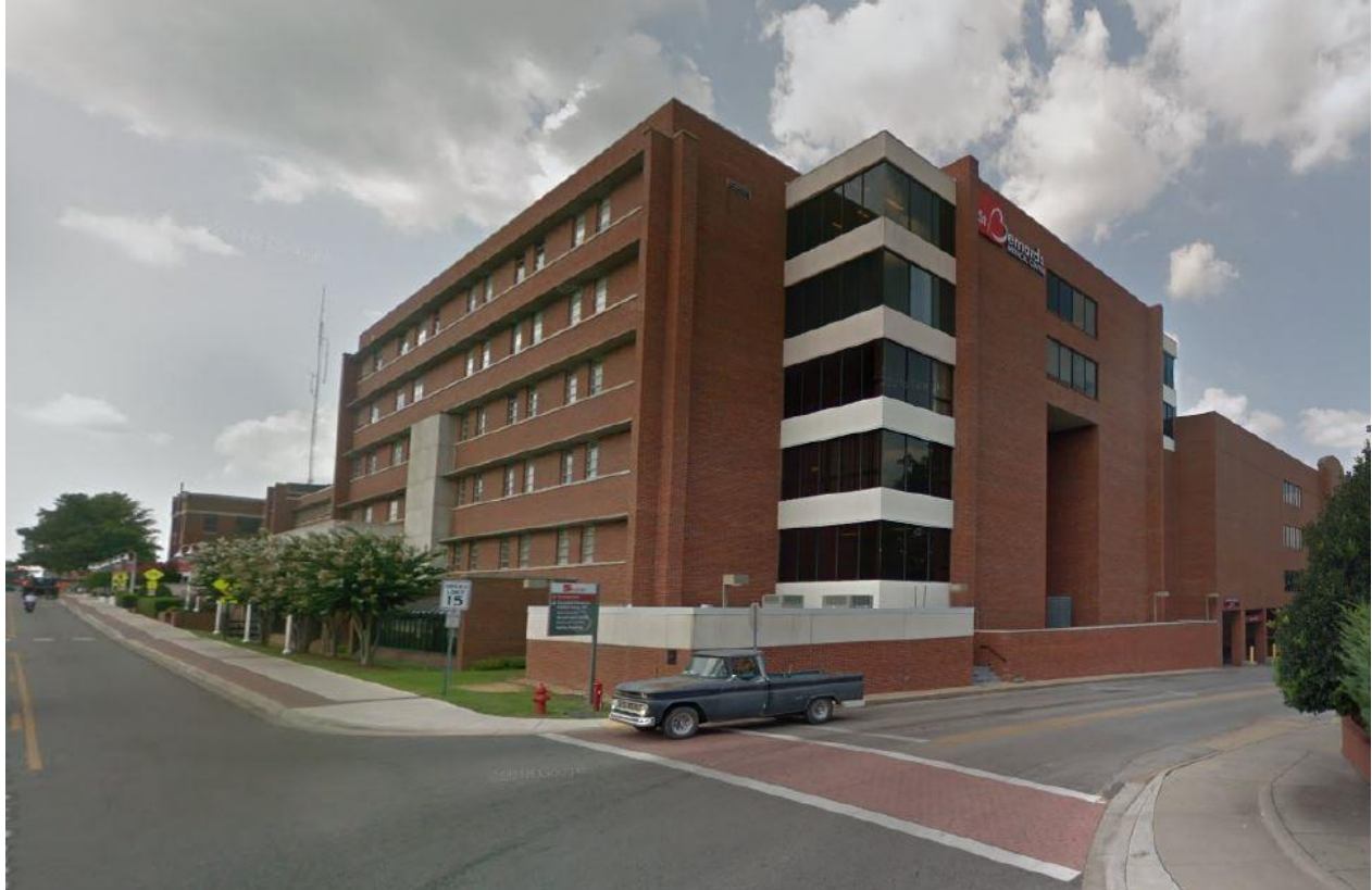
St. Bernard's Hospital, East Wing, east side View is looking northwest from E. Matthews Ave and Carson St Picture Source: Google Street View
