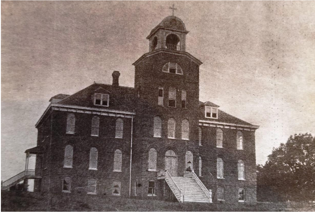
East side of 1898 Convent, view is looking west.
