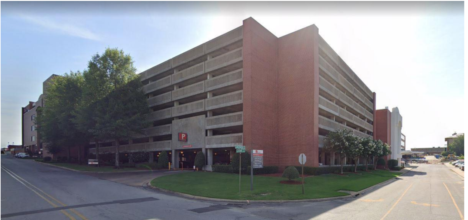
St. Bernard's Parking Garage View is southwest at corner of E. Jackson Ave & Carson St Picture Source: Google Street View , northeast corner
