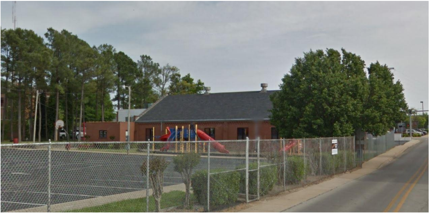
Blessed Sacrament Parish Hall, north side View is southeast from S. Church St. Picture Source: Google Street View
